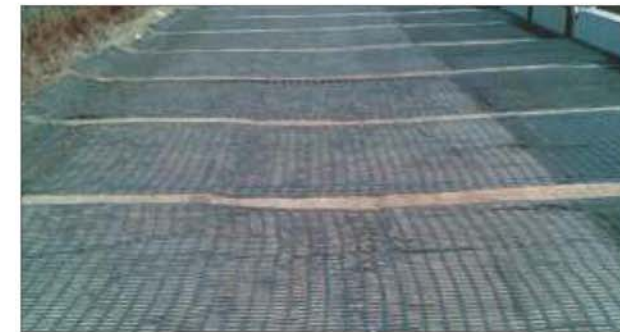
Step 5: Placement of StrataGrid
