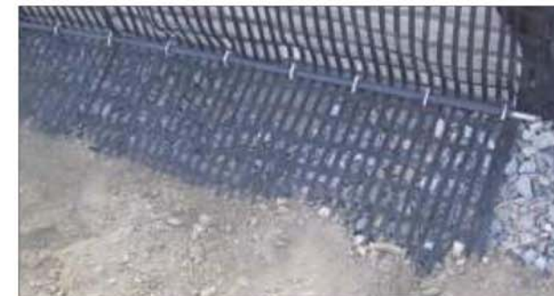
Step 7: Installation of StrataGrid
