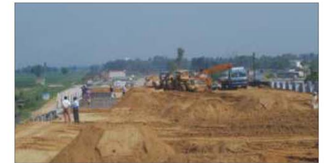
Step 6 : Grading of Backfill
