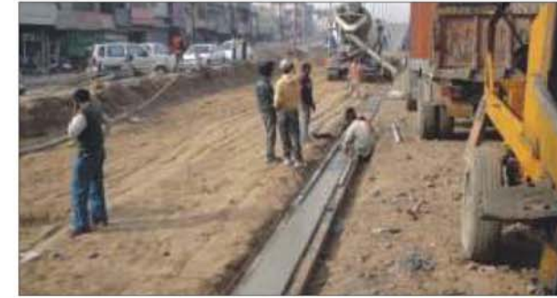
Step 3: Casting of Levelling Pad
