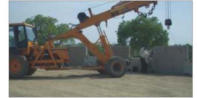
Step 4 : Place StrataWall on Levelling Pad
