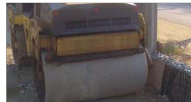
Step 9: Compaction of Soil
