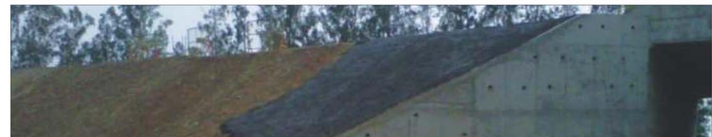
Step 7: StrataWeb geocell treated & finished slope surface
