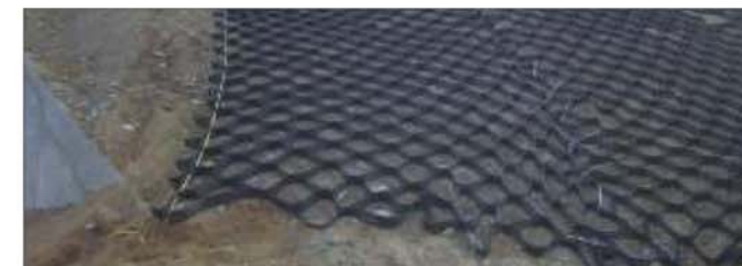
Step 3: Install the StrataWeb section in the designated portion using necessary expansion and anchoring
