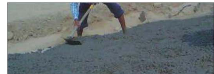
Step 6: Compaction and dressing of the finished slope surface
