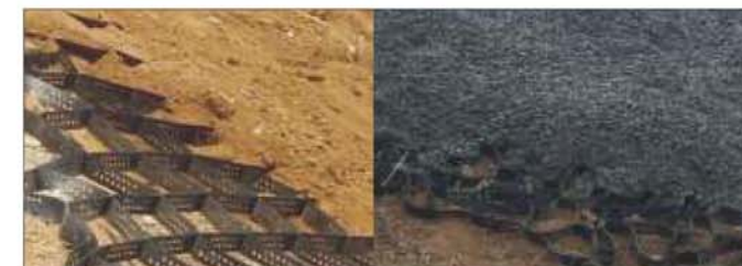
Step 5: Infilling of StrataWeb geocells with necessary infill material
