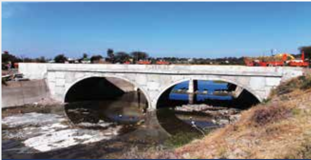
Multi-span bridge over Bhima canal on NH-9, Pune - Solapur
