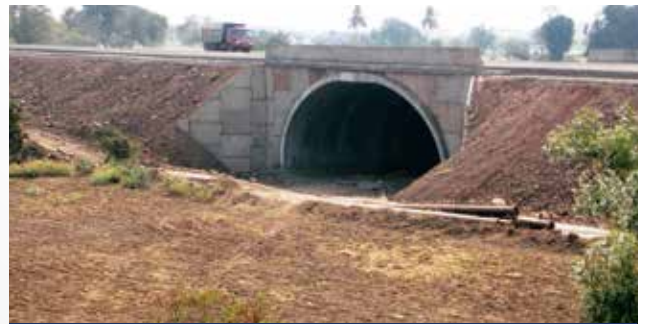
Bridge over Tembhorni bypass on NH-9
