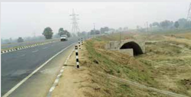
Arch over live gas pipeline on NH-30
