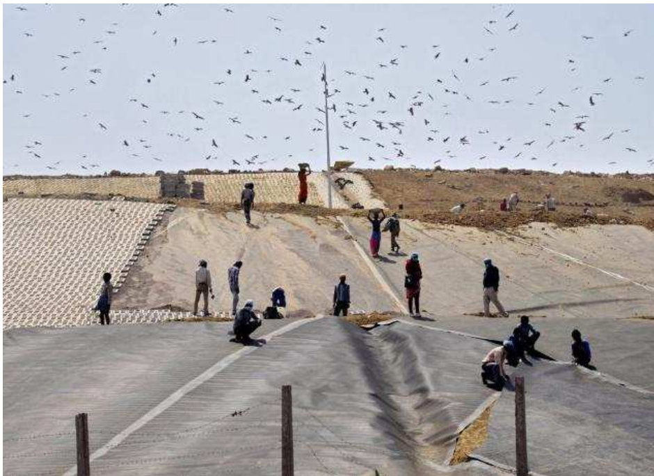
East Delhi Municipal Committee workers covering the garbage with geo grids and geo sheets at the Ghazipur landfill site near the Delhi-Uttar Pradesh border. Photo: Rajeev Bhatt
