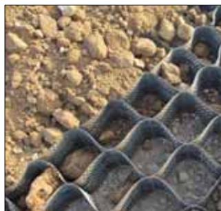
Fig 1: Typical Geocell
