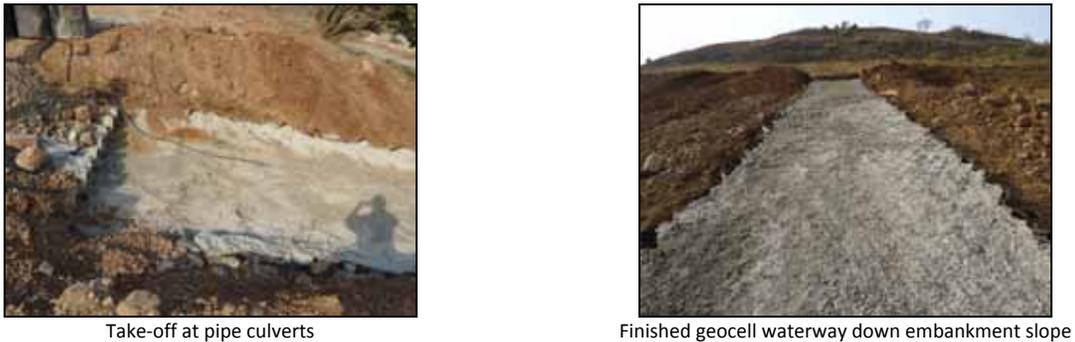
Fig. 7: Waterway along road embankment slope
