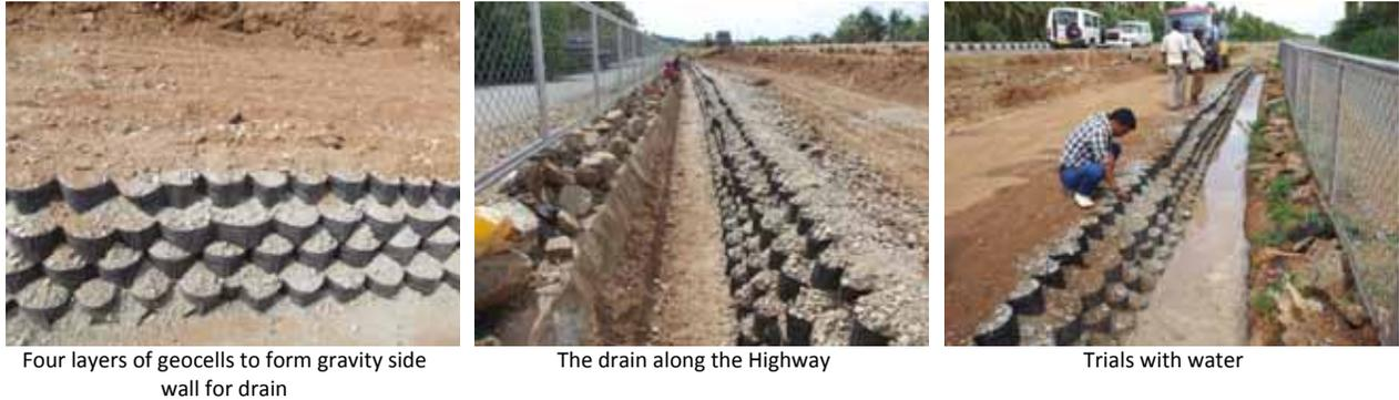
Fig. 6: Trial stretch of side storm water drain along NH-4
