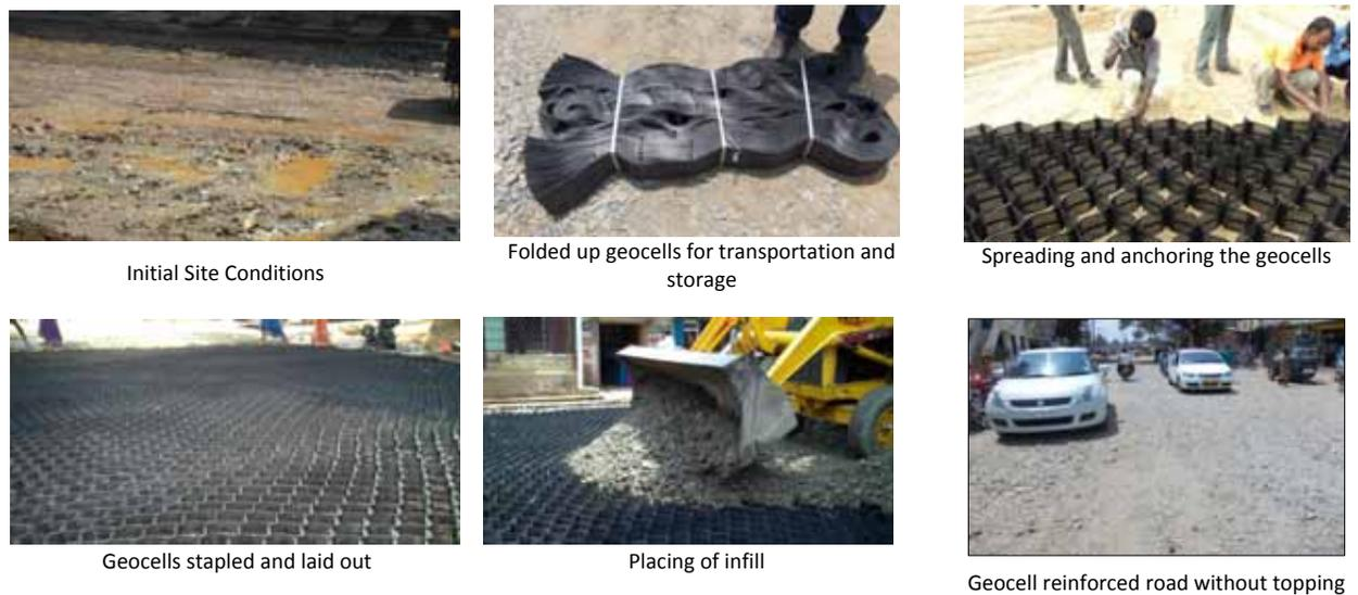
Fig. 3: Sequence of road rehabilitation
