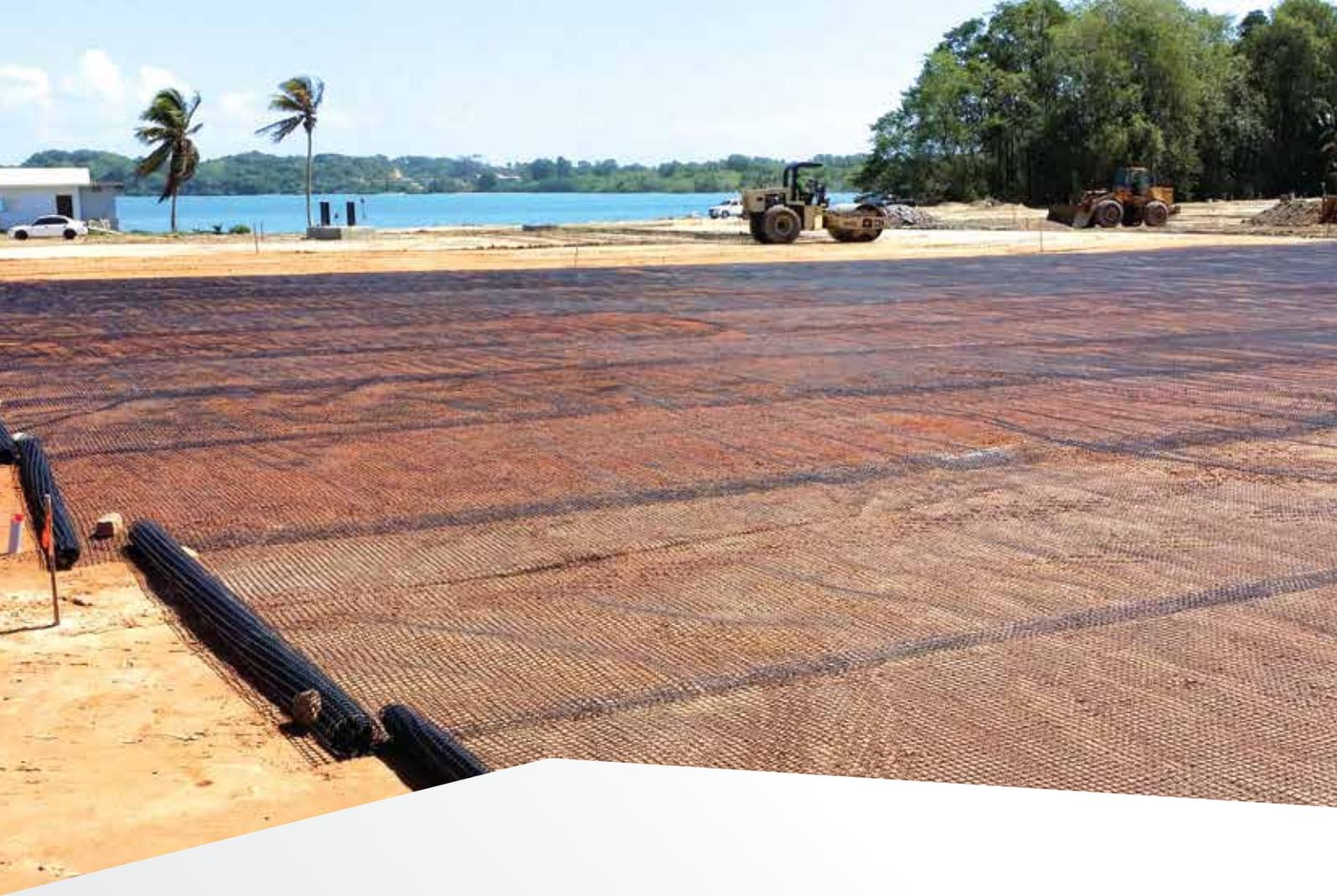
StrataBase is an extruded, polypropylene, rigid biaxial geogrid. It functions as structural reinforcement within paved and unpaved road sections, and at the base of embankments on weak soils, through superior junction strength and interlocking aperture stability.
