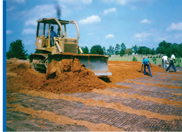
Fill is placed atop StrataGRID in the Reinforced Structured Slope.
