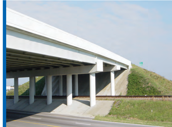
The completed Clemson Road bridge abutment.
