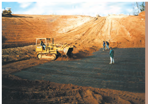
STRATAGRID lies flat for easy installation.
