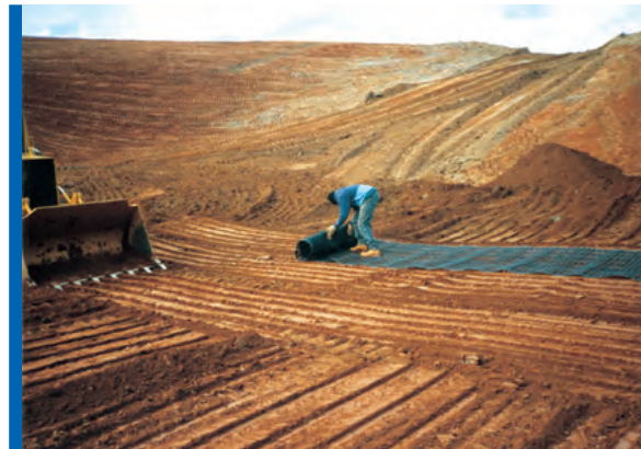
Subgrade is graded flat in preparation for STRATAGRID placement.
