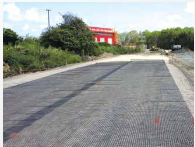
Stabilization of haul roads
