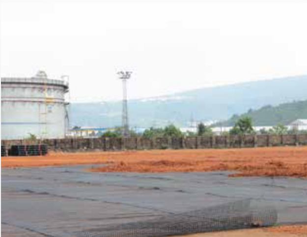
Subgrade and foundation improvement
