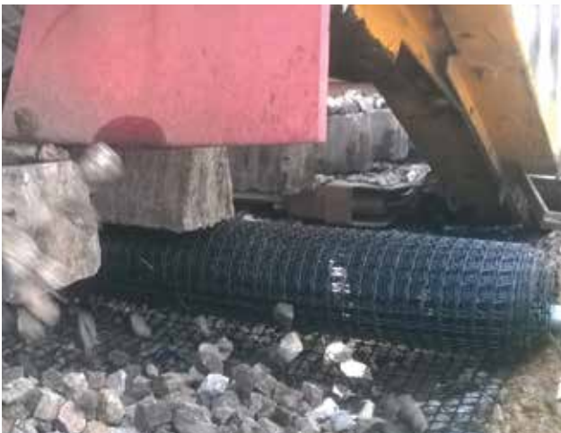
Ballast & sub ballast stabilization
