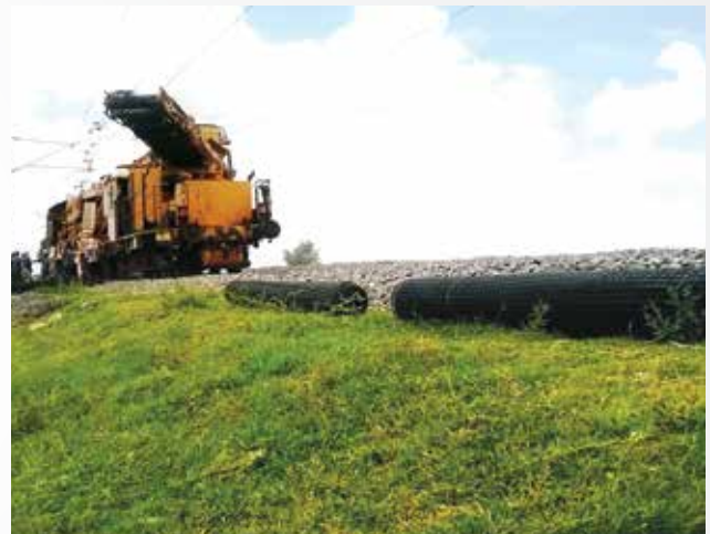
Railway track bed stabilization
