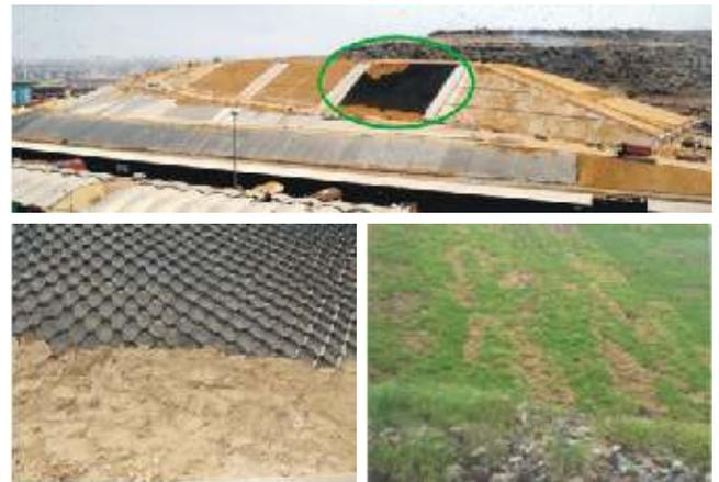
Fig. 4: Landfill Project near Delhi; example of turfing with StrataWeb
