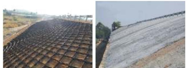
Fig 3: Highway embankment – NH 202; example of facilitating placement of pcc with StrataWeb
