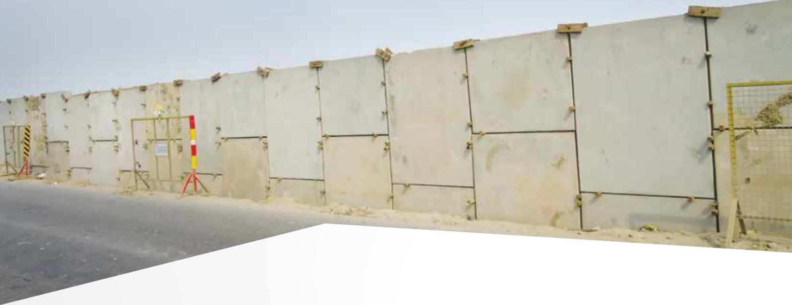
StrataWall™ is a precast concrete panel wall fascia for a reinforced soil structure. StrataWall™ is designed to give a positive concretion with StrataGrid™ geogrids as a reinforcing material.
