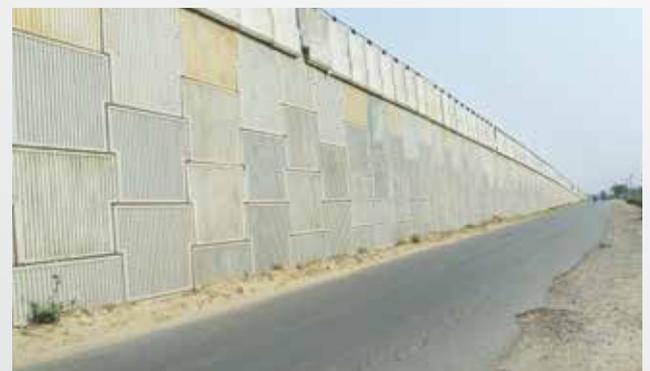
RS Wall with precast reinforced concrete panels
