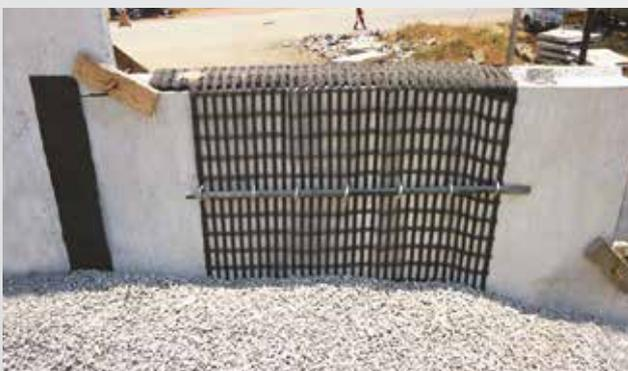
Arrangement of StrataGrid™ reinforcement with panels
